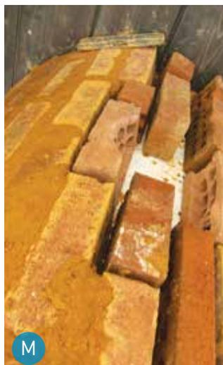
» **If you used a metal armature**, cut a hole in the mesh, then attach the chimney to the armature and lay the final bricks around it.
