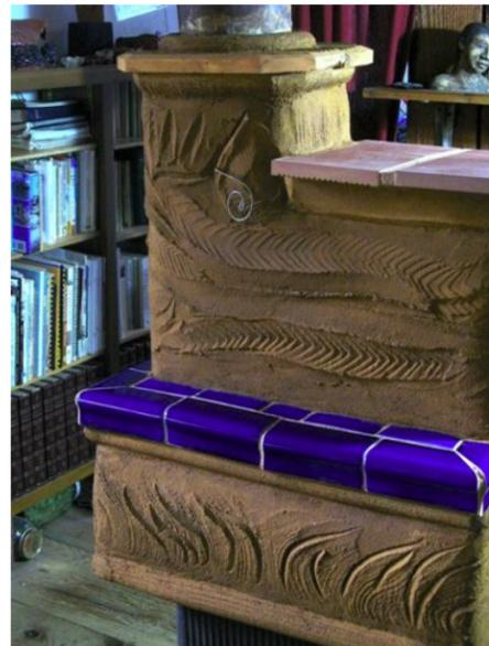
On cracking: most of the cracks are vertical. Three of them extend from level 2 to level 4, one each at the corners, and one in the middle. The middle crack continues up through the next level — that's the widest one. The horizontal crack is at level 4, from the bottom L up to the bottom of the flat red tile.
